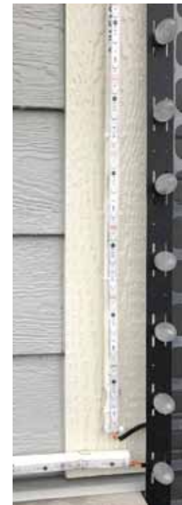
House C9 Outlines - Strawberry C9s from holidaycoro. - Used on roofline, garage, front door, and each window net frame. - Gutter clips used for gutters and roof. - C9 Strips used for garage and front door from Boscoyo Studio.
